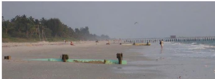
Figure 1-3. Typical Outfall Blockage (Outfall 9)
